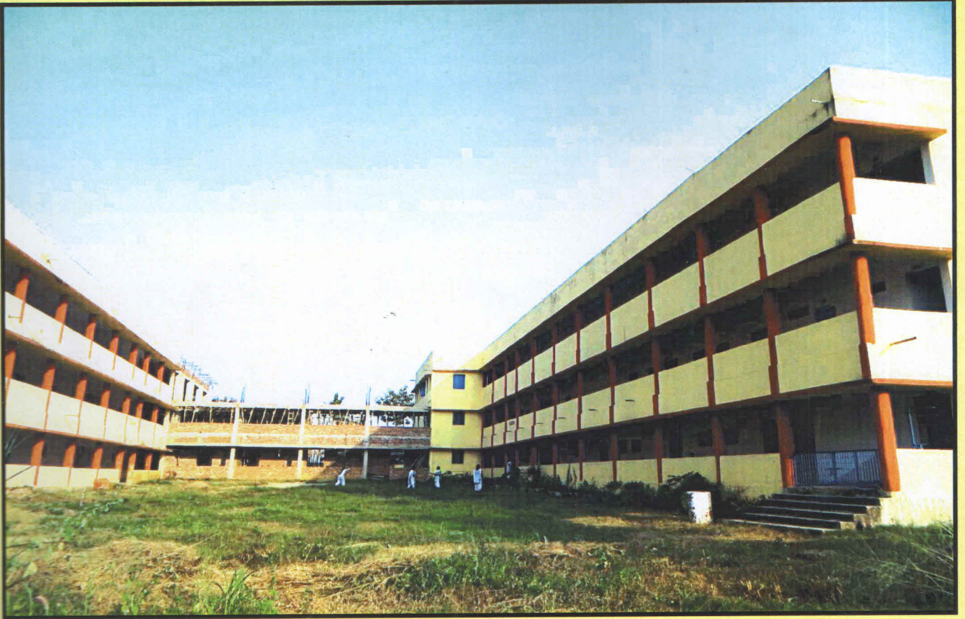
Building of Al-Habeeb Teacher's Training College Sector - VI, Bokaro Steel City - 827006 (Jharkhand)
